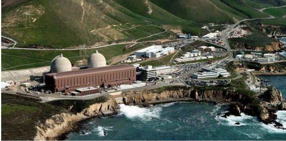
Diablo Canyon Nuclear Power Plant
